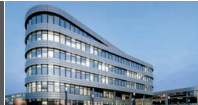
Smoke extraction RheinEnergie AG, Cologne, Germany 4
